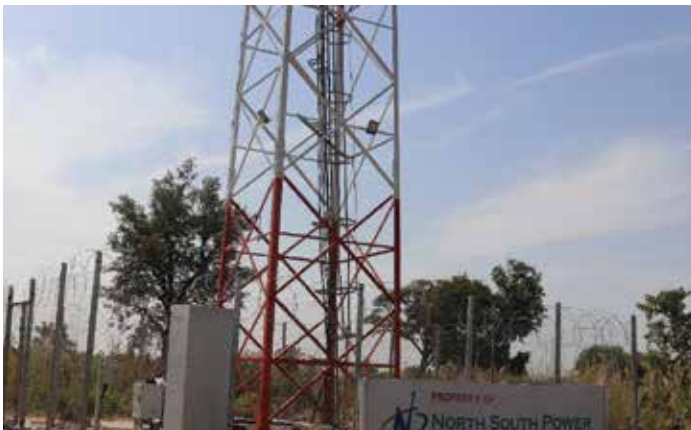
NSP COMMUNICATION MAST (SIDE VIEW)
