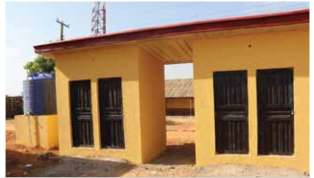
ZUMBA SCHOOL PROJECT TOILET FACILITY
